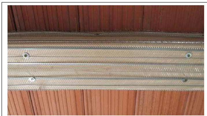
Figure A.7.3: Detail of the mesh fixing.
