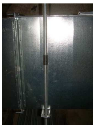
Figure A.6.1: Ductwork hanging system and METU-System transversal joint.
