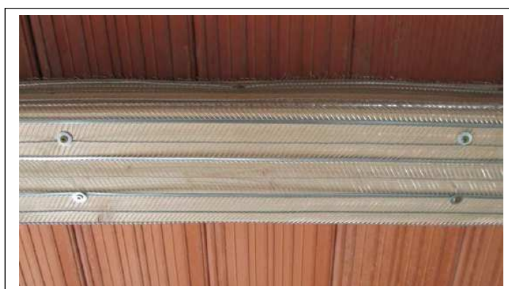
Figure A.7.3: Detail of the mesh fixing.
